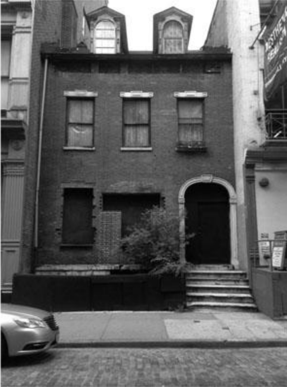
FIGURE 8.1 The only remaining building on the Greene Street block from the 1820s–1850s residential era. (Author’s photo, 2013.)
